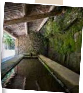
Lavoir / Wash house
